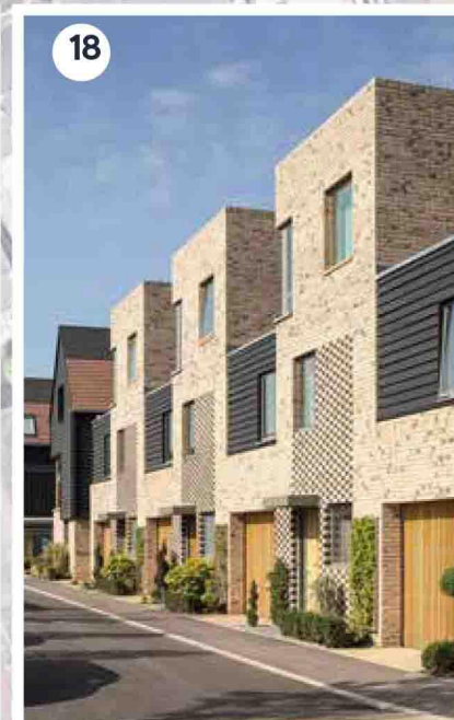
Streets with integral parking, Winchester Street
