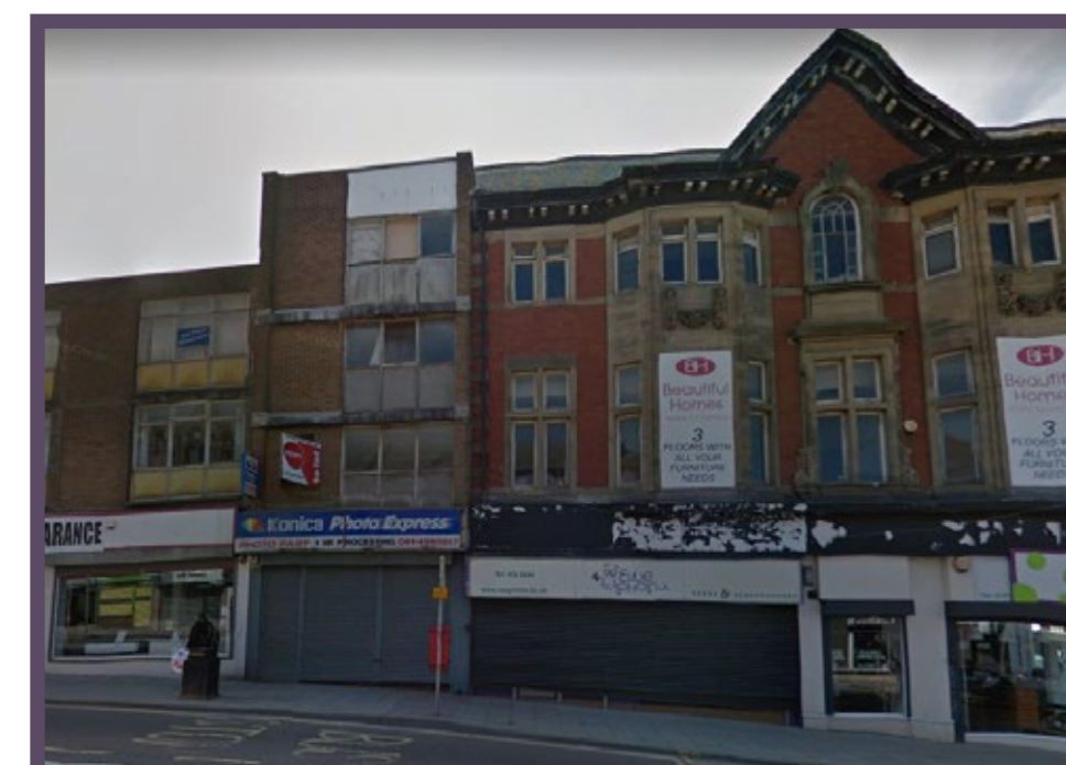
Vacant buildings detract from the appearance of the area
