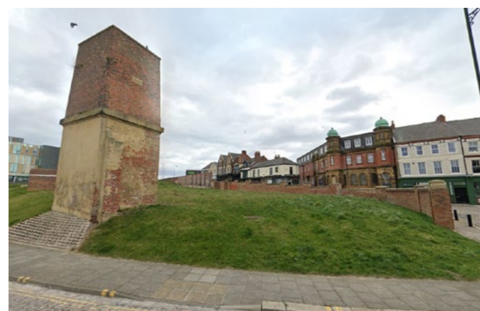
Former Glassworks chimney
