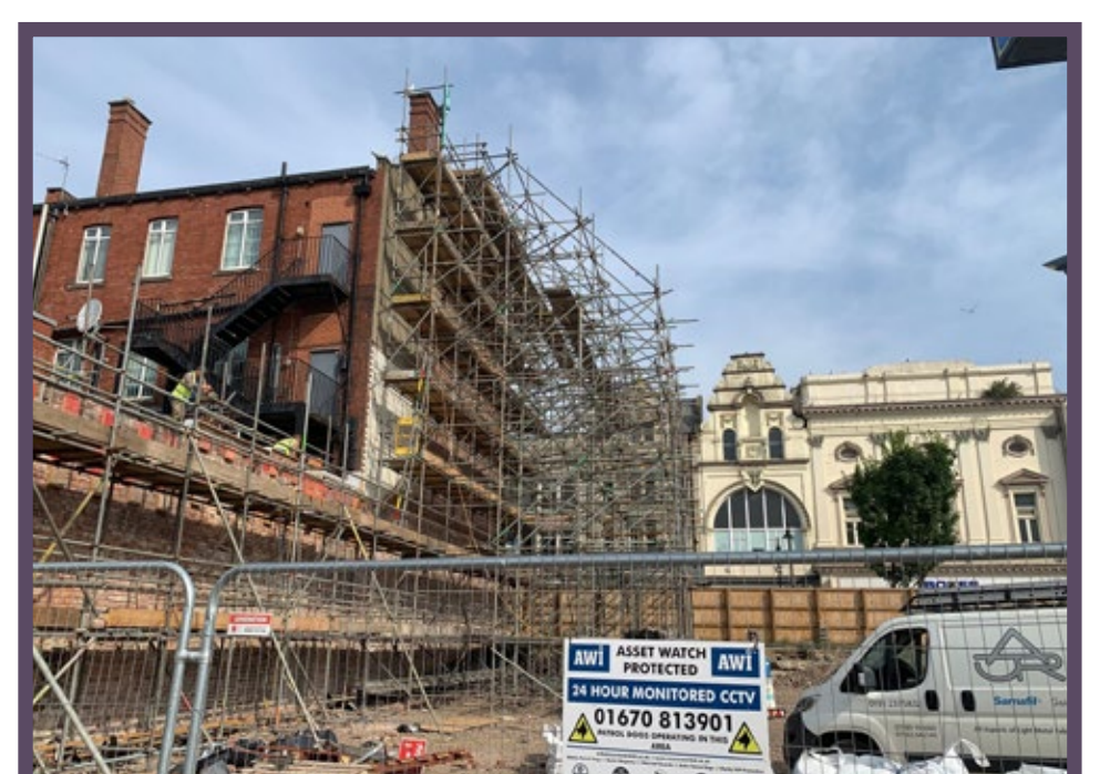
Scaffolding to gable of Lloyds bank building on King Street
